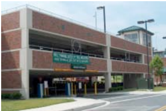
Longwell Parking Deck is capable of adding another level of parking
